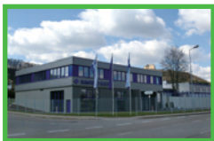
1 Sumitomo Electric Hartmetallfabrik GmbH
